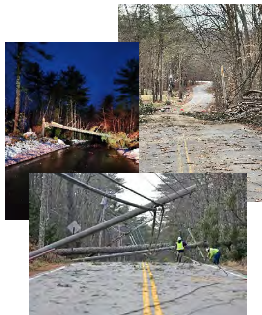
Figure 1 - Storm Damage NH
